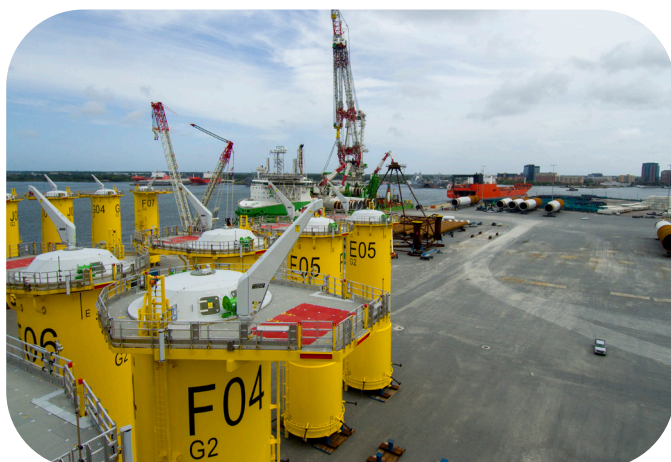
PORTSMOUTH MARINE TERMINAL: Portsmouth Marine Terminal is being repurposed to handle large offshore wind components for Dominion Energy's Coastal Virginia Offshore Wind project, creating a valuable site for deployment of future development across the region.
