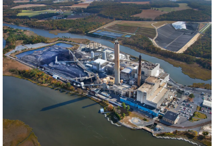
The former Indian River Power Plant in Sussex County, Delaware, where offshore wind energy from US Wind would come ashore and connect to the regional grid. Credit: Delaware Business Times
