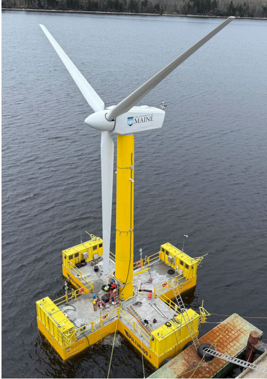
The University of Maine's quarter-scale floating offshore wind turbine moored off Castine is the most advanced floating wind prototype ever tested in U.S. waters. Credit: University of Maine
