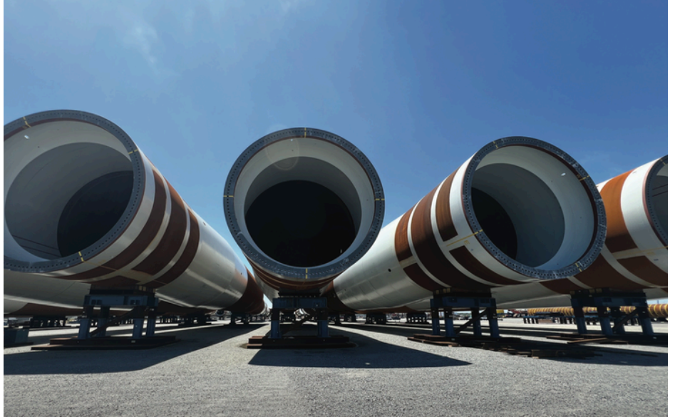
Massive steel foundations at Portsmouth Marine Terminal await their trip offshore to become part of Dominion Energy's 2.6 gigawatt wind project off the Virginia coast. Credit: Oceantic Network
